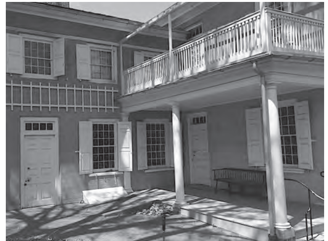
Deshler-Morris House (Germantown White House), Philadelphia residence of George Washington.
