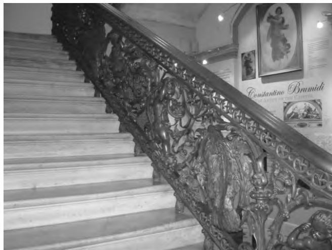
Cast-iron decorative stair rail on staircase in Senate hall of the Capitol.
